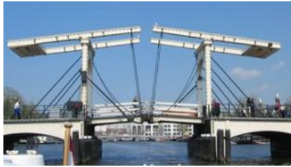
Meager Bridge (Amsterdam)
