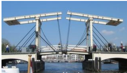
Meager Bridge (Amsterdam)
